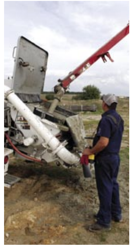
Pump to pump operation is monitored using Schwing's Vector Control System which provides valuable two-way communication between pump and operator.
