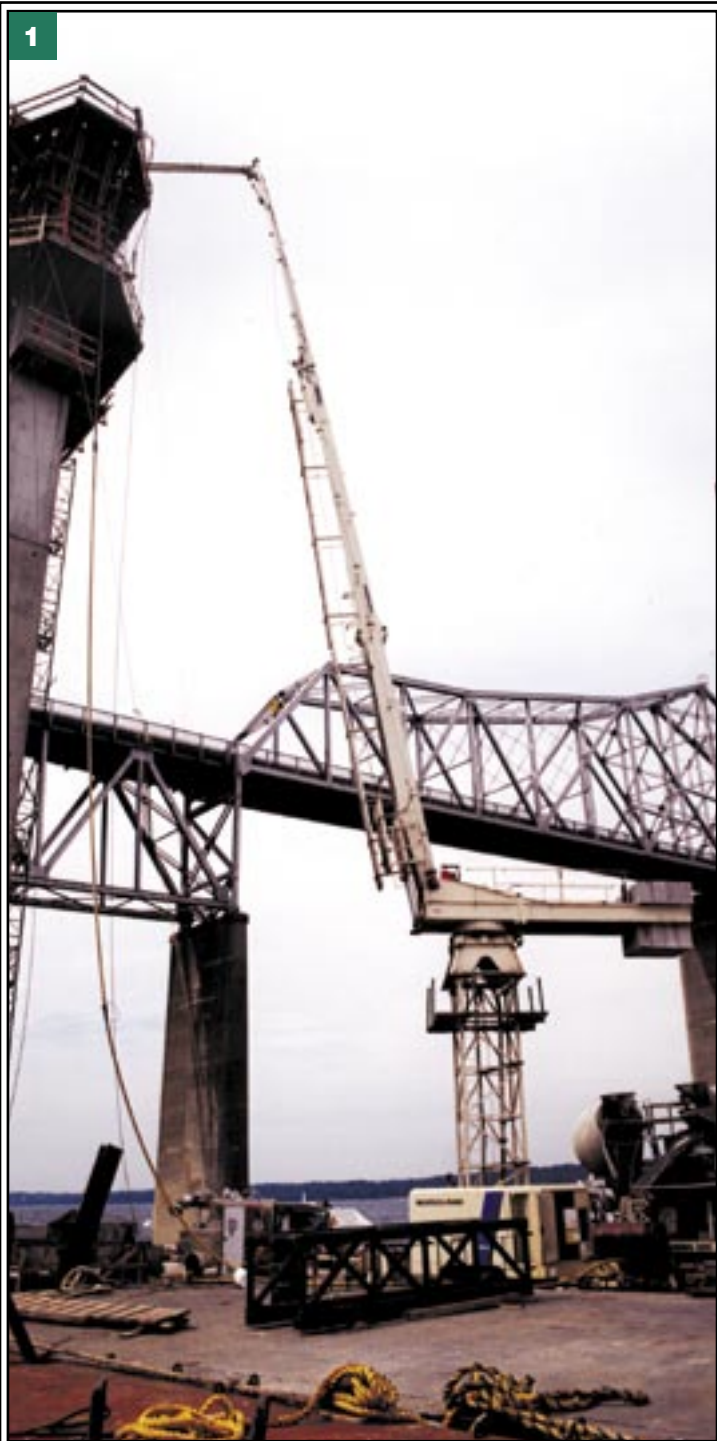
1. DVM 42-meter boom mounted on a lattice tower places substructure concrete on Rhode Island's Jamestown Bridge.
